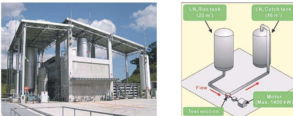
Fig.1 Cryogenic Inducer Test Facility (CITF) at Kakuda Space Center (KSC)
