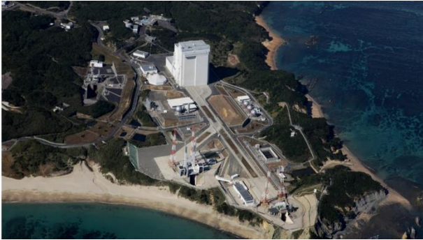
Fig. 9 Tanegashima Space Center launch complex
