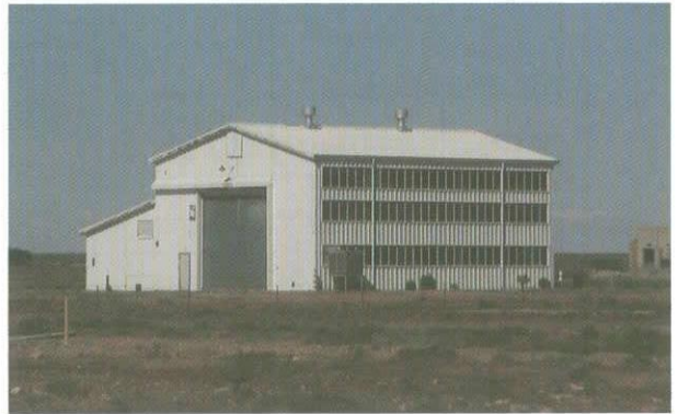
図3.13-9 EFS(Explosive Fitting Shop)
