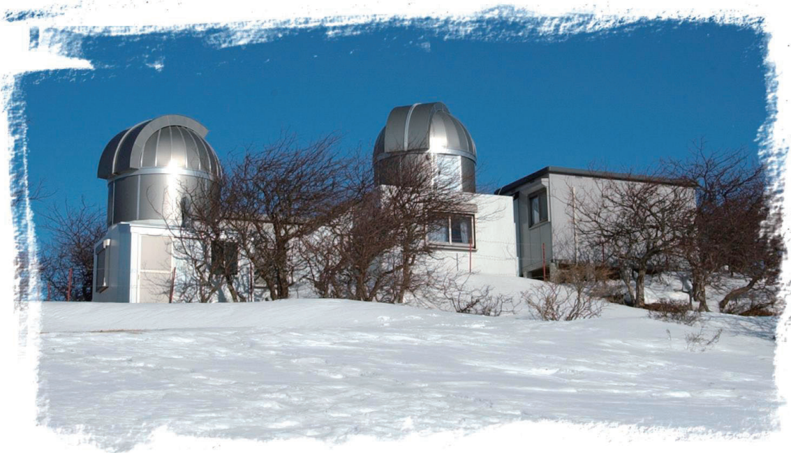
Overview of the facility
