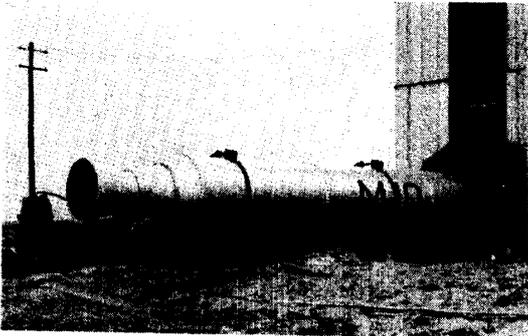
FIG. 30. Mu rocket engine for the ground static test.
