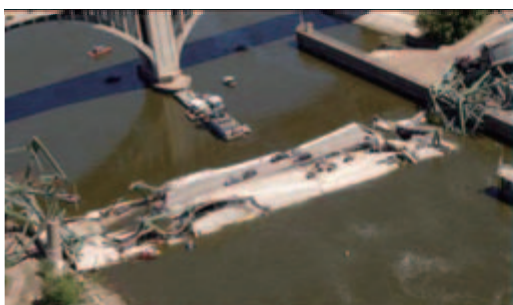
Collapsed highway bridge in Minnesota Accident report, National Transportation Safety Board, http://www.nts.gov
