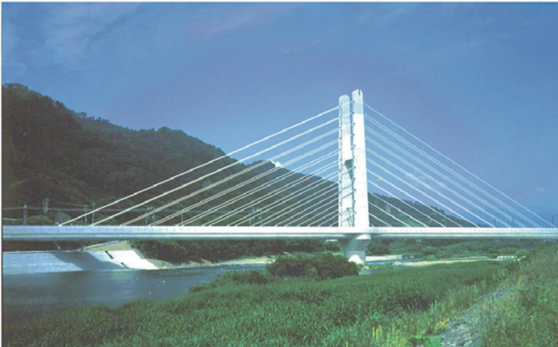
Cable-stayed long-spanned concrete bridge (Length 270m, Height 96m)
