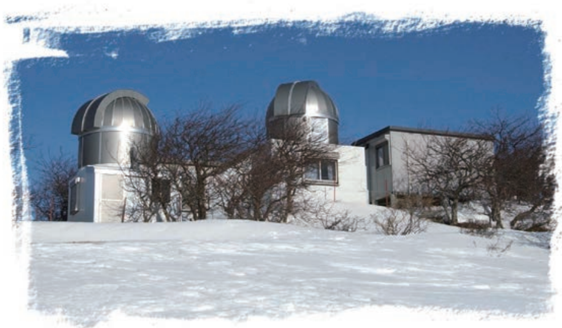
Overview of the facility
