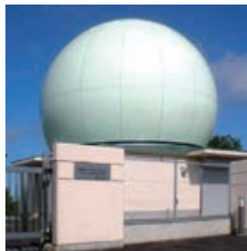
Phased array radar of Kamisaibara space guard center
