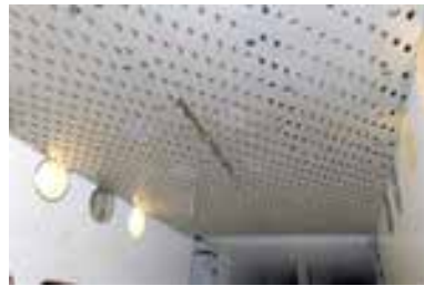
Figure 14: Top wall (with a pressure rail).
