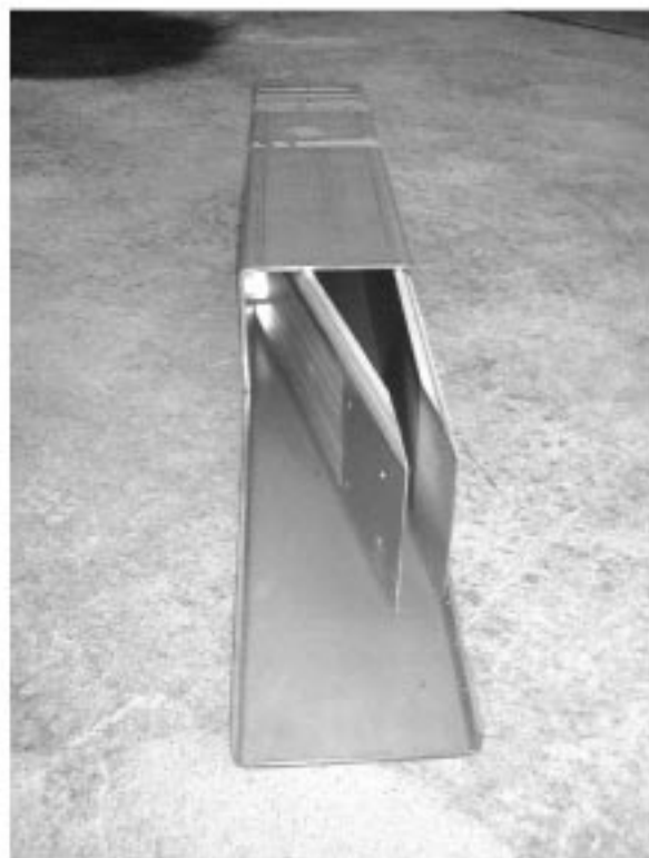
Fig. 3.2.9 A mishap due to starting load in the M3.4 wind tunnel: the 20 mm thick aluminum plate in the diffuser was bent in the wind tunnel starting.
