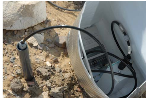
Fig. 3 Soil moisture measurement device
