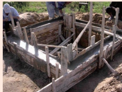
Sensor Hut Construction
