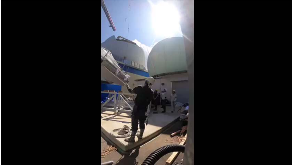
Transmitter hanging operation
