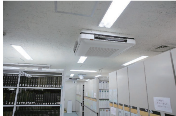
Renewed air-conditioner at ISAS Library
